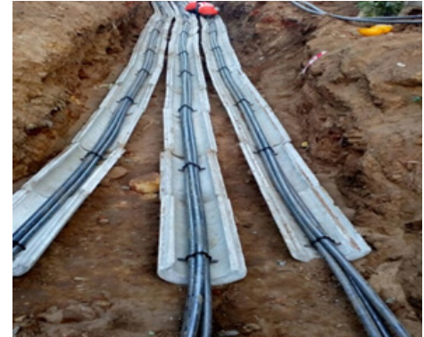
Figure 11 Pre-fabricated half-cut Hume pipes (Typical trench)
