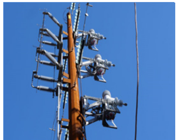
Figure 21 Sub-Transmission Recloser
