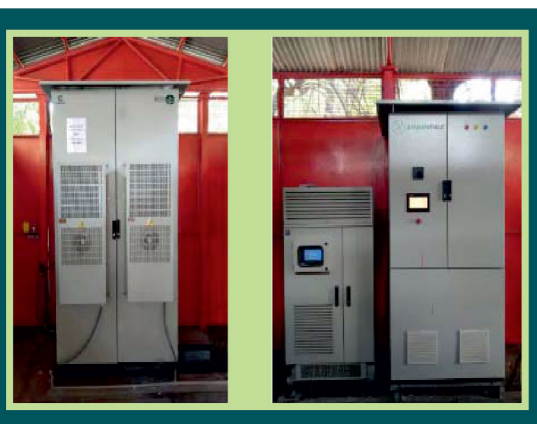
Figure : From left, Battery enclosure, PCS / Inverter and ACDB / EMS enclosure
